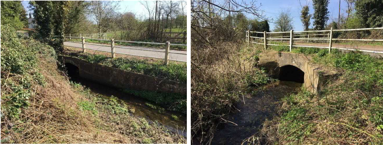
Figure 2-2: Photographs upstream (left) and downstream (right) of existing Cantley Lane South culvert
